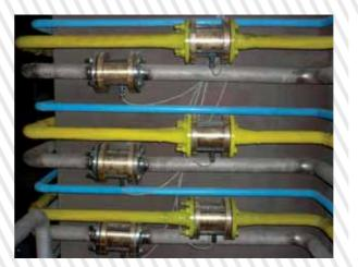
The principle of intervention is based on a PT100, that is indirectly hit by a rise in temperature, which modifies the value of the resistance. This resistance difference is elaborated by PLC, which generates an alarm signal. The detect time is 2 sec.
